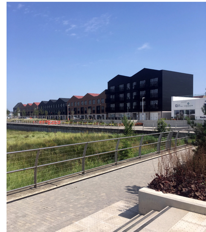
Waterfront residential uses, walkways and reed beds at Rochester Riverside.
